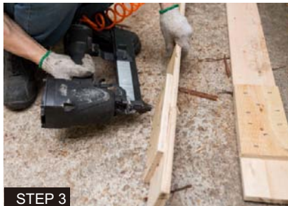
STEP 3 Encompass the countertop with slats and attach them with a nail gun.
